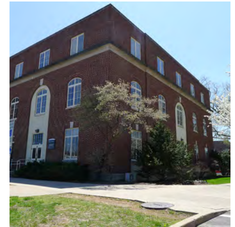
Northeast Exterior Corner of Reber
