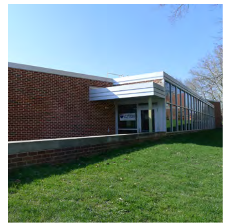
Entrance to Engineering Services
